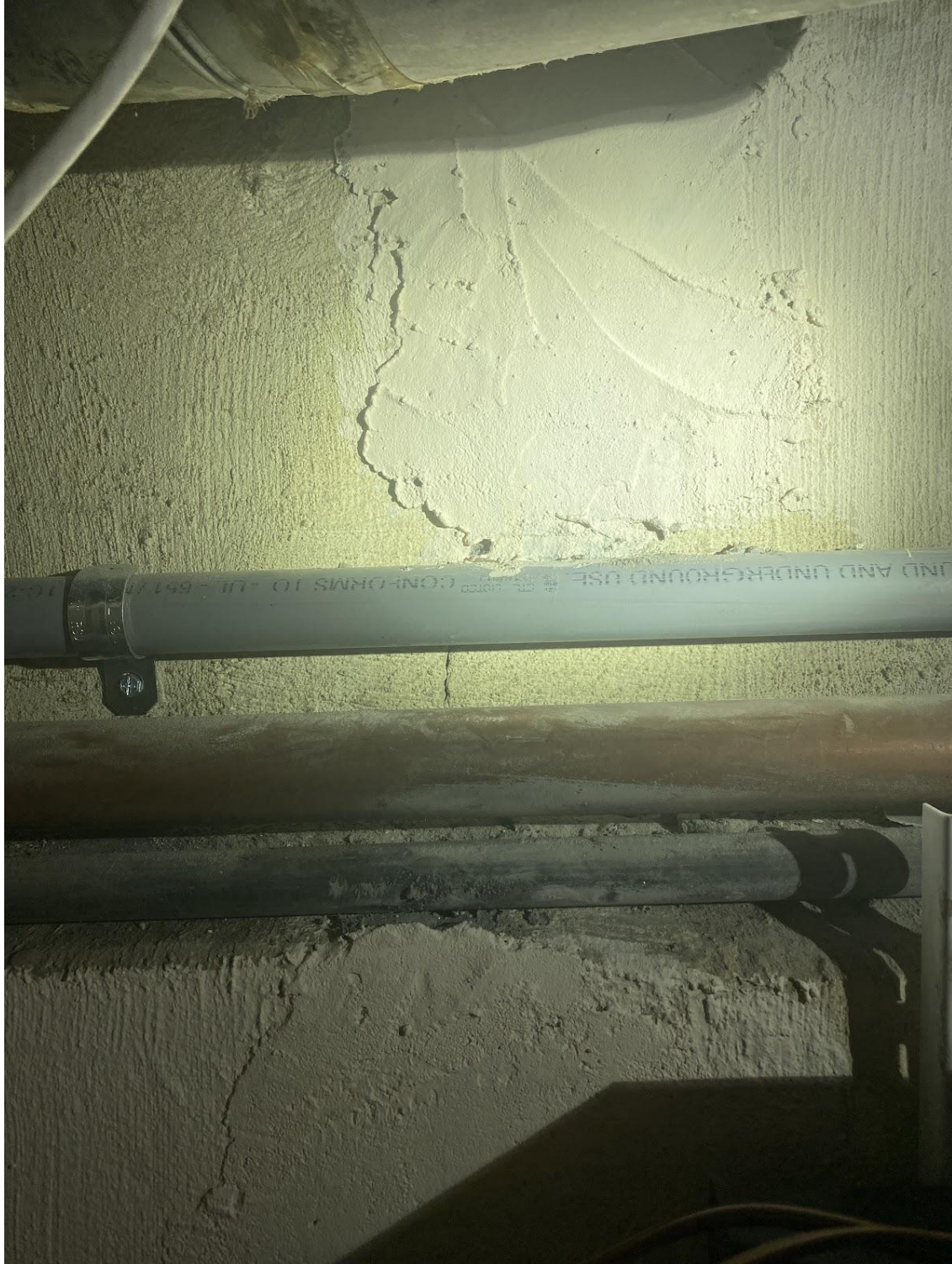
Vertical crack with patching. No crack through patch material.
