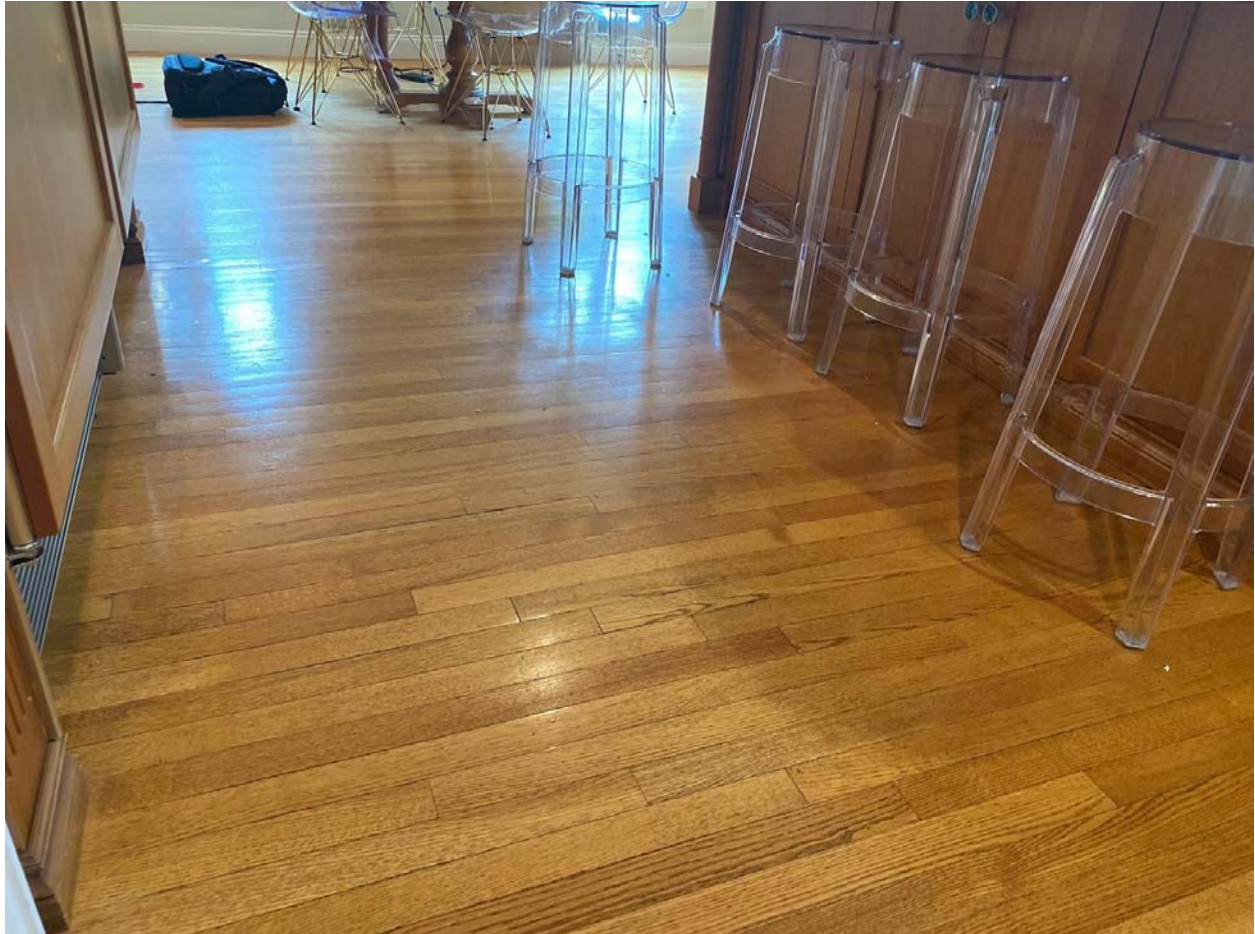
Kitchen floor area with minor interior settlement.
