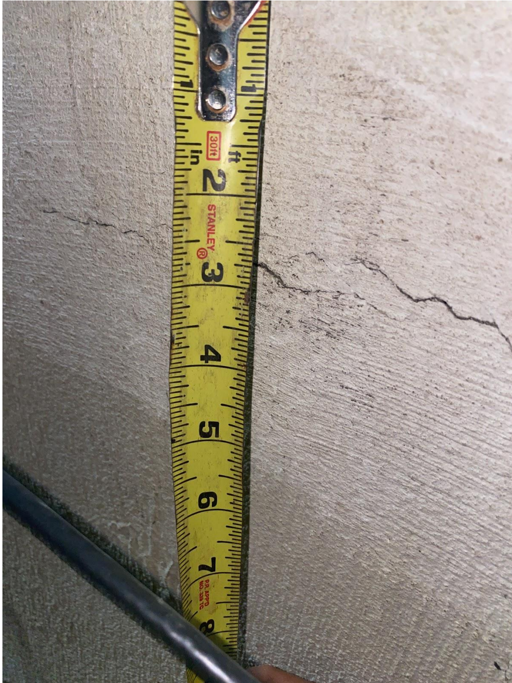
Close-up of horizontal crack.
