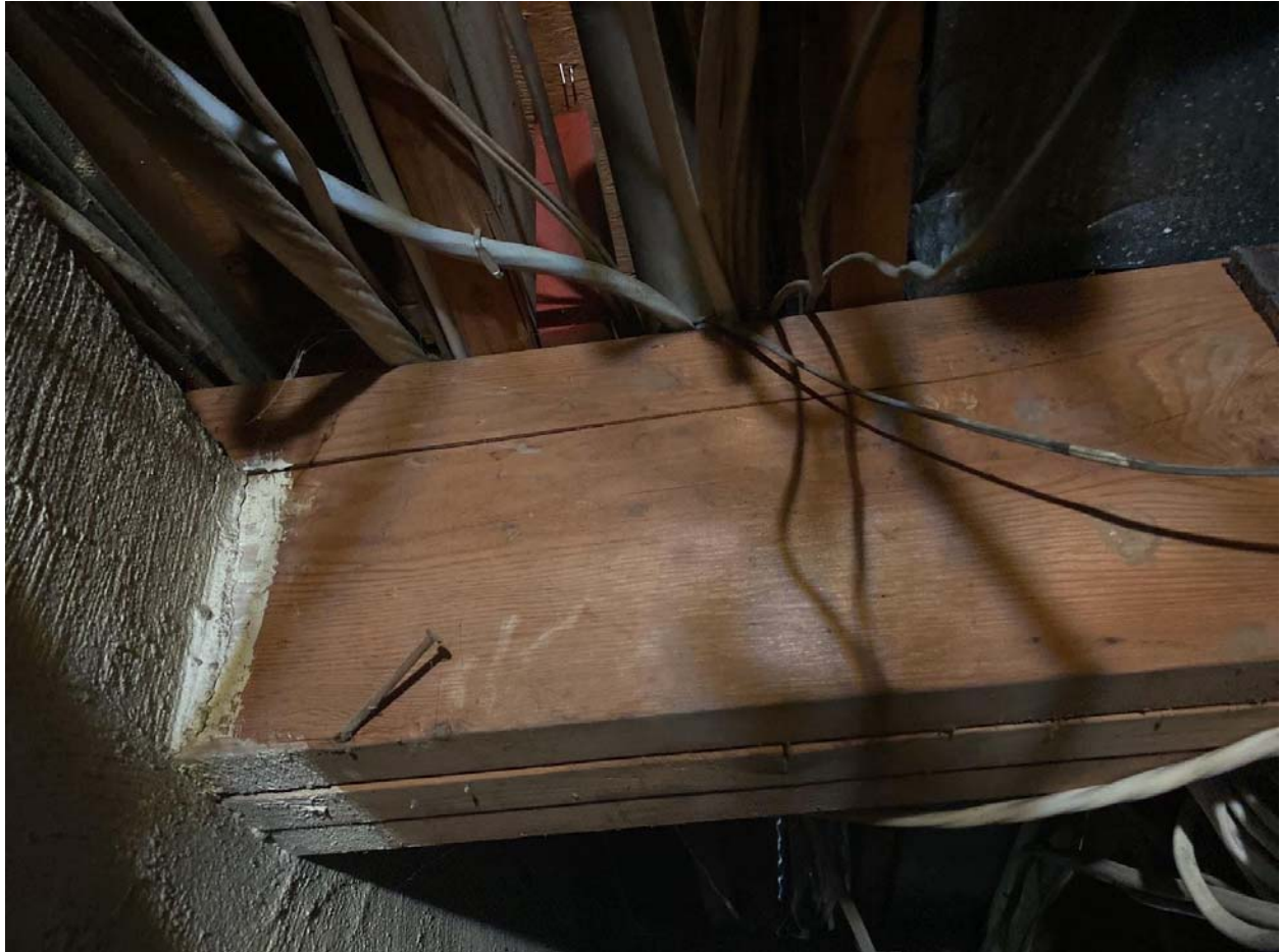
Main support beam with crack near top on front most layer.
