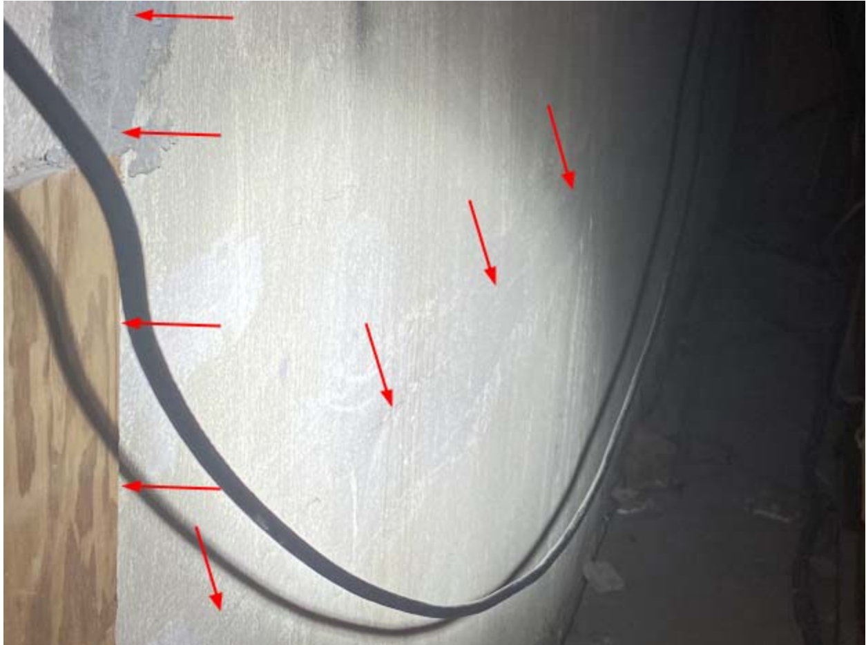
Vertical and horizontal cracks meet near the front of left foundation wall.
