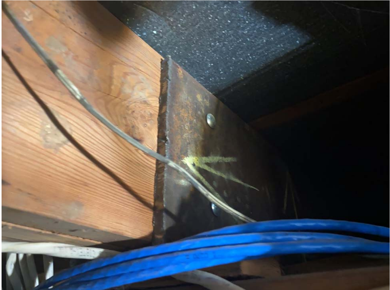
Main beam with Steel plate bolted on (similar steel plate on opposite side).
