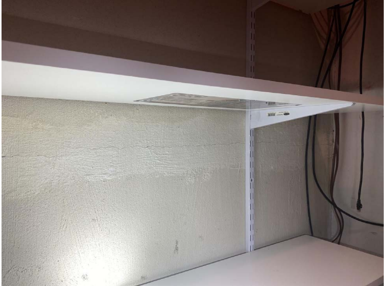
Horizontal crack with patching / painting in closet area towards rear of home.
